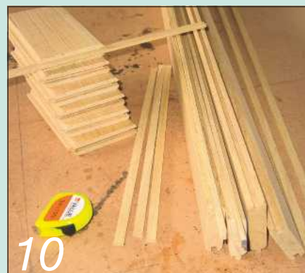
10 A few strips were required as an extra tongue on some of the boards
