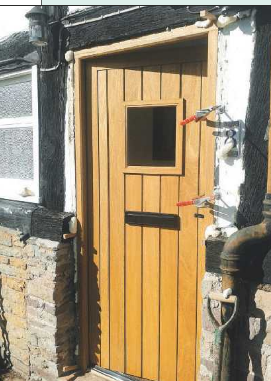
Now the recesses in the outer frame can be cut to take the locking points
