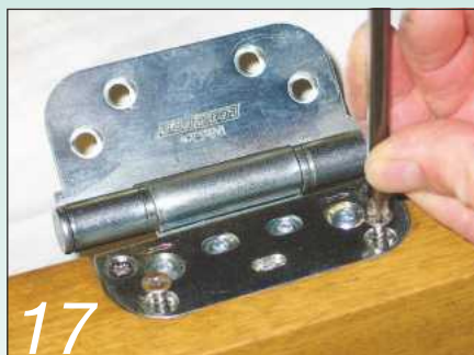
The fully adjustable hinges can now be fitted in their recesses in the outer frame
