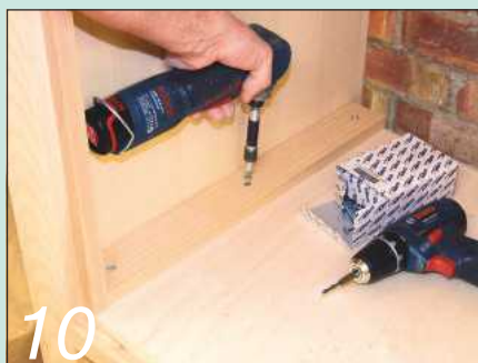
10 Fit two offcuts of wood at each side of the shelf to act as oven guides
