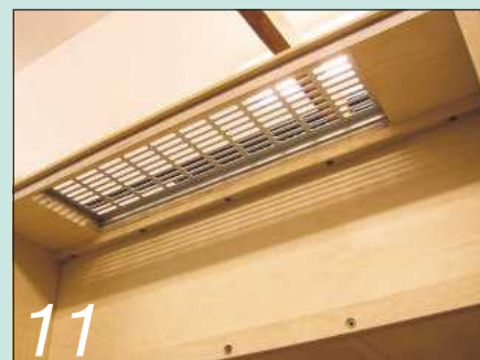
11 Mark the position of the opening for the top ventilation grill and cut it out
