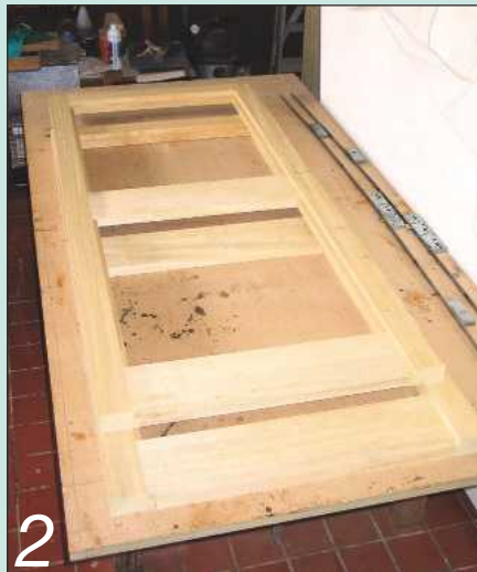
2 The frames for the two doors each consist of two stiles and three rails
