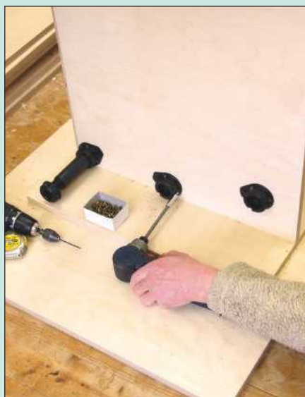
2 Hold the carcass corner joints square using plywood webs and cramps
