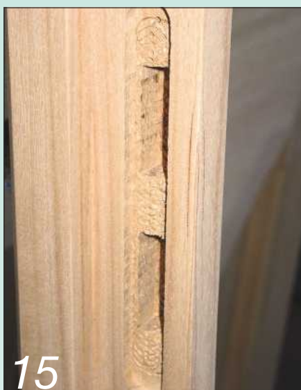
Now the recesses in the outer frame can be cut to take the locking points
