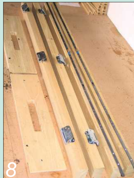
8 All the door components have now been fettled to take the furniture
