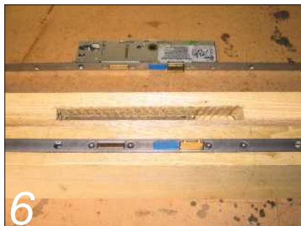
6 The three-point locking system drops into full-length slots and recesses
