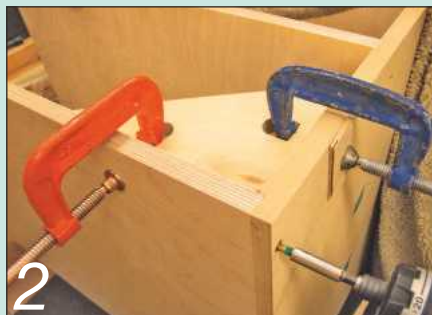
2 Hold the carcass corner joints square using plywood webs and cramps
