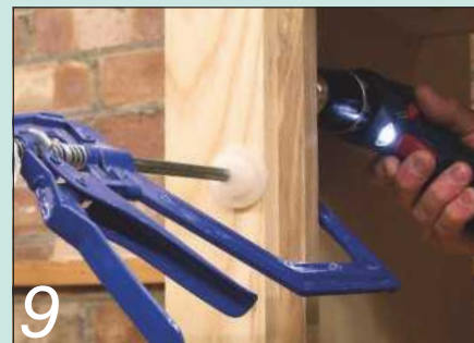
9 Attach strips of ash to the inside of the face frame for the oven fixing screws
