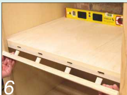
6 Dry-fit the face-frame rail to the edge of the oven shelf using floating tenons
